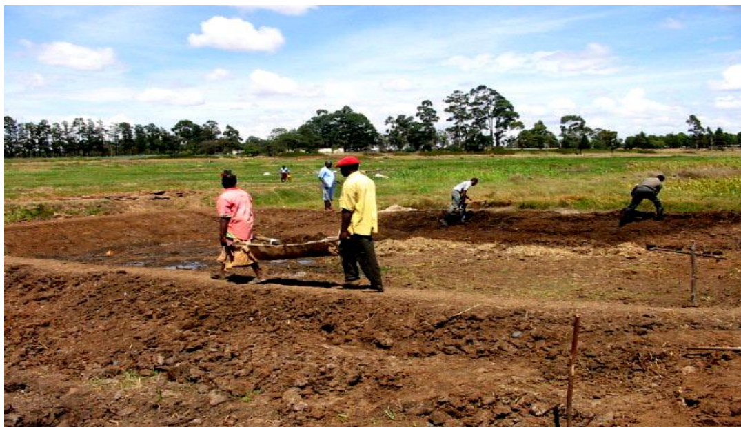
Figure 2: Use of manual labour in fishpond construction in Kenya
