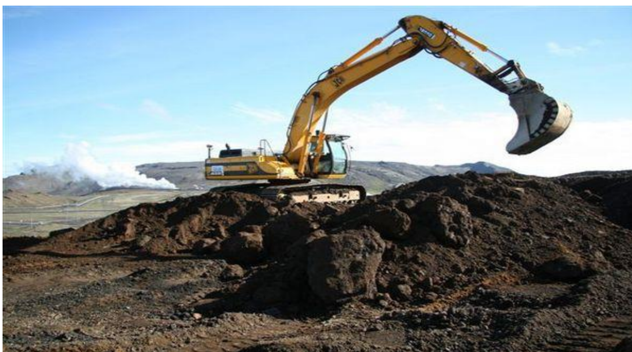
Figure 4. Rock and soil materials at Gígahnjúkur were mixed and spread to imitate the natural texture and create a good condition for vegetation colonization (Photo: Námur.is, 2017)
