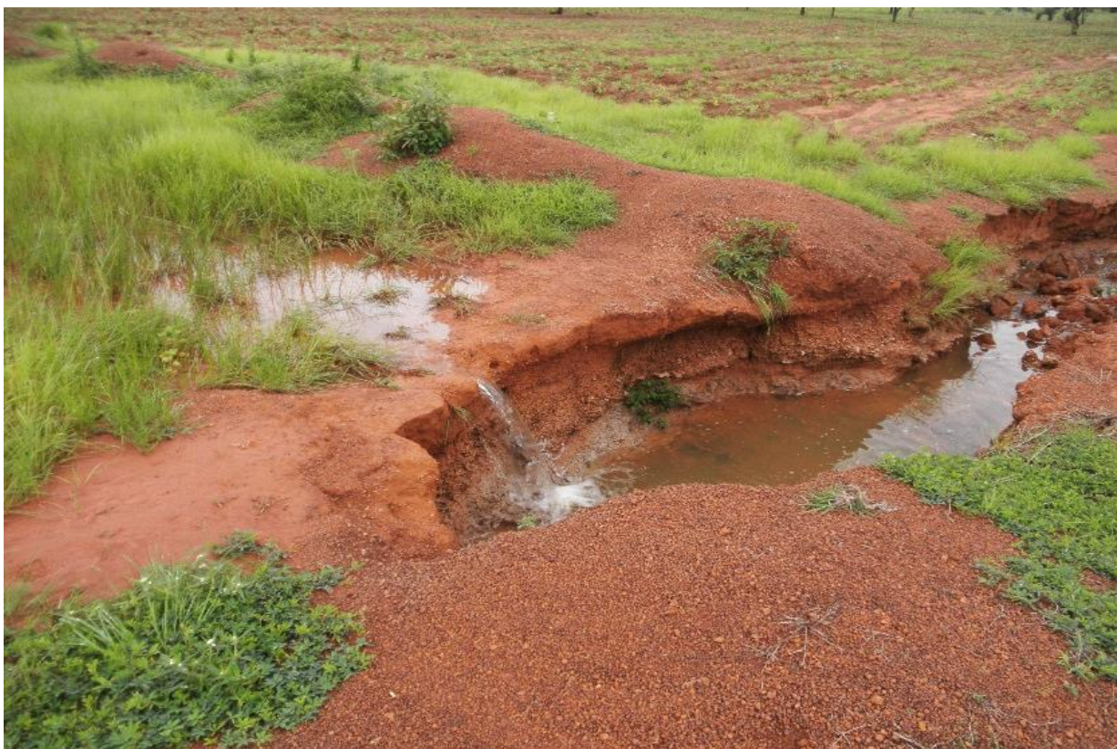
Figure 6. Gullies formed on farmlands adjacent to the mine site. This gully on Hafiz' farmland is in the path of the runoff from the mine (Photo by Awal Rashid, 7 th July 2016).
