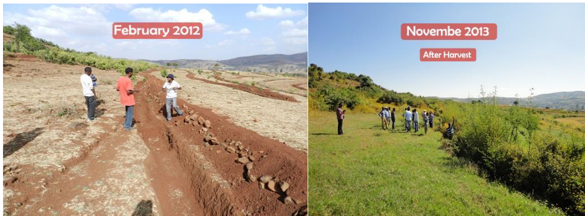
Figure 8. Rehabilitated landscape in Debre Yacob watershed. Photo on the left is a baseline photo just after the construction of physical SWC measures. Photo on the right is taken one and a half years later, after the physical structure was reinforced with biological measures (Photo: WLRC).
