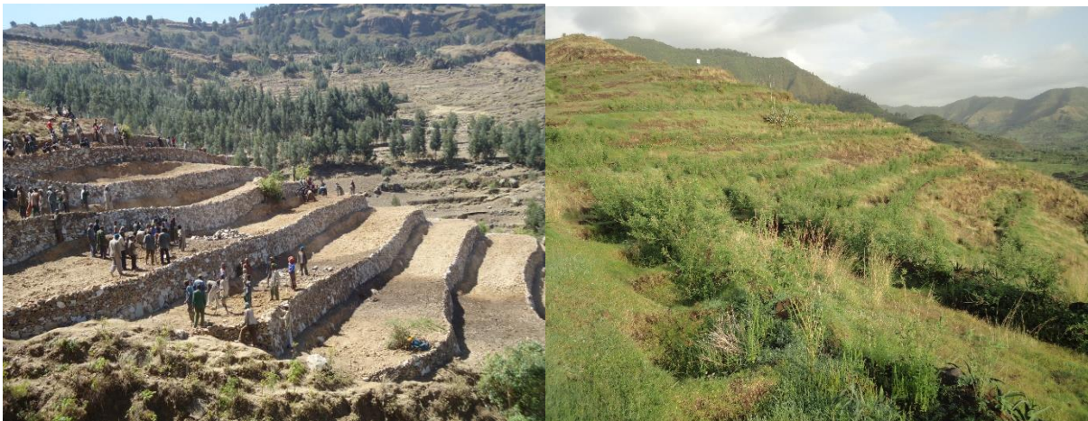
Figure 5. Land rehabilitation efforts of the government program in the highlands of Ethiopia. Left photo shows community effort on the construction of a bench terrace in Meket Woreda, North Wollo Zone. Photo on the right shows rehabilitated watershed using both physical and biological measures, Habru Woreda, North Wollo Zone (Photos: Aytnew E. Tatek 2012).
