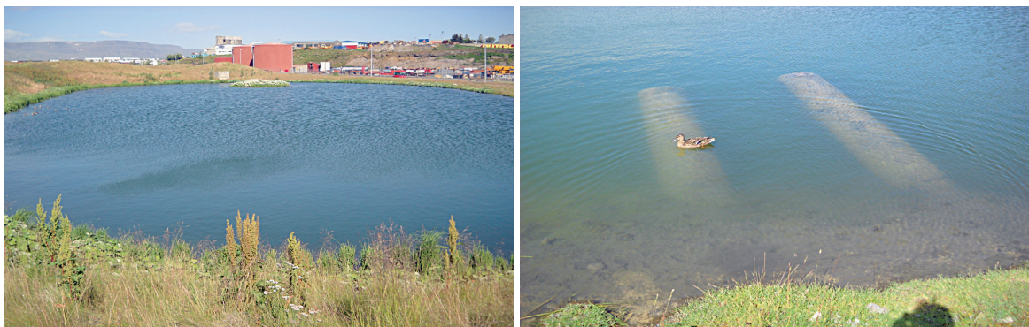
Fig. 7. Wastewater sediment treatment pond along the River Ellidaá; the pipes channel water from wastewater drains/channels to the pond for settling and then drainage into the river.
