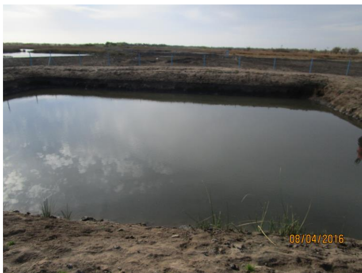
Figure 5: The effect of pond erosion (run off) in some of the fish ponds in CRR.
