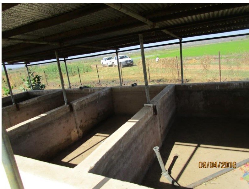
Figure 6: The side view of non-functional nursery tanks at National Fish Hatchery in SAPU CRR.
