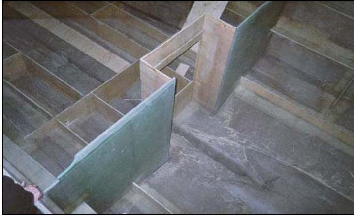
Figure 8: Watertight bulkhead in construction.
