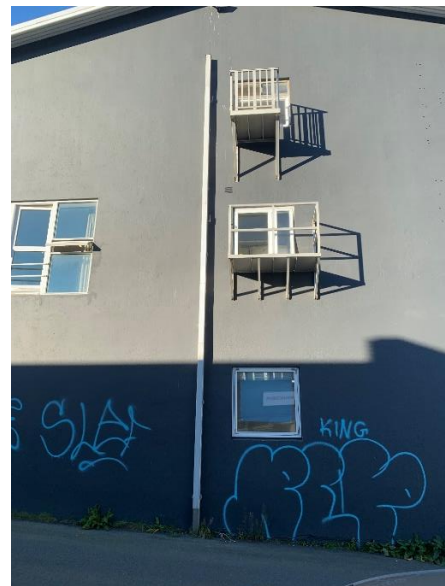
Figure 14 Emergency exit and ladder
