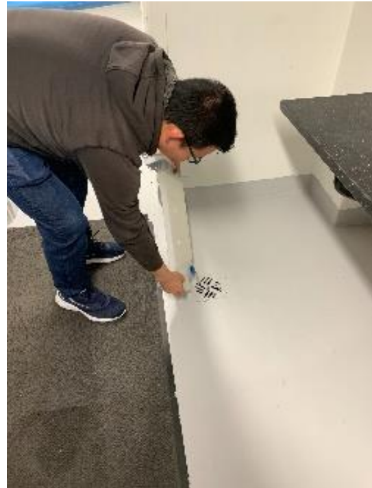
Figure 7 Water to be poured down the drain on the floor.
